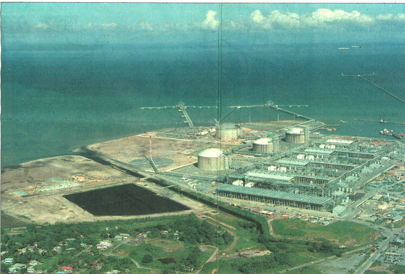
PHOTO COURTESY OF EMERSON PROCESS MANAGEMENT
